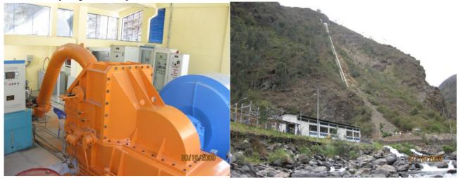
Sandia hydropower plant is situated in far southeastern Peru in Puno province, 15km to Sandia downtown. It is a small run-of-the-river type with an installed capacity of 1200kW and a water head of 220m, and it is also the first Pelton project for Hangzhou Yatai awarded in overseas market.
