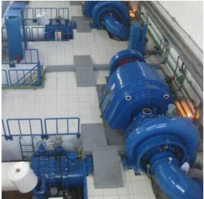
Invested by H.G.M. Enerji Inş. Nak. Gıda Güb. Yem San. ve Tic. Ltd. Şti., Keklicek hydropower project is at suburban area of Malatya in the southeast of Turkey. The water head of the power plant is 166m and it consists of 2 horizontal Francis turbine-generator units with total installed capacity 2×4337kW. Hangzhou Yatai supplies the electro-mechanical equipment and achieves the acceptance and commercial commissioning in July 2009.
