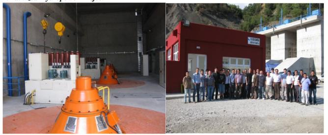
Yalnizca hydropower project involves the construction of a 15 MW (consisting of 3×5MW vertical Kaplan turbines with double regulating performance). It is developed by Filyos Enerji Uretim ve Ticaret A.S. The project is located 10km southwest of the city of Karabuk, along Filyos River (or "Filyos Cayi") in Karabuk province, in the west Black Sea region of Turkey. This power plant including a computer-based control system is put into the commercial operation in September 2009.
