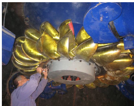
Runner installation for four-jet Pelton turbine
